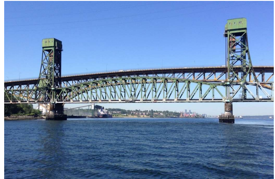
A view of the vertical lift on CN's Second Narrows Bridge in Vancouver's Burrard Inlet. The growth in both rail and marine traffic has already heightened congestion problems on this vital piece of transportation infrastructure. Completion of the Trans Mountain Pipeline is expected to result in a more than 50% increase in the number of ships moving under the bridge. (Image courtesy of Mark Hemmes)
