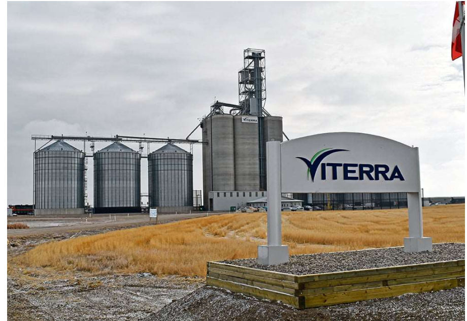
A view of the Viterra grain elevator located in Lethbridge, Alberta, one of many Canadian facilities to be acquired by Bunge Limited through a potential merger of the two companies. (Image courtesy of The Western Producer)
